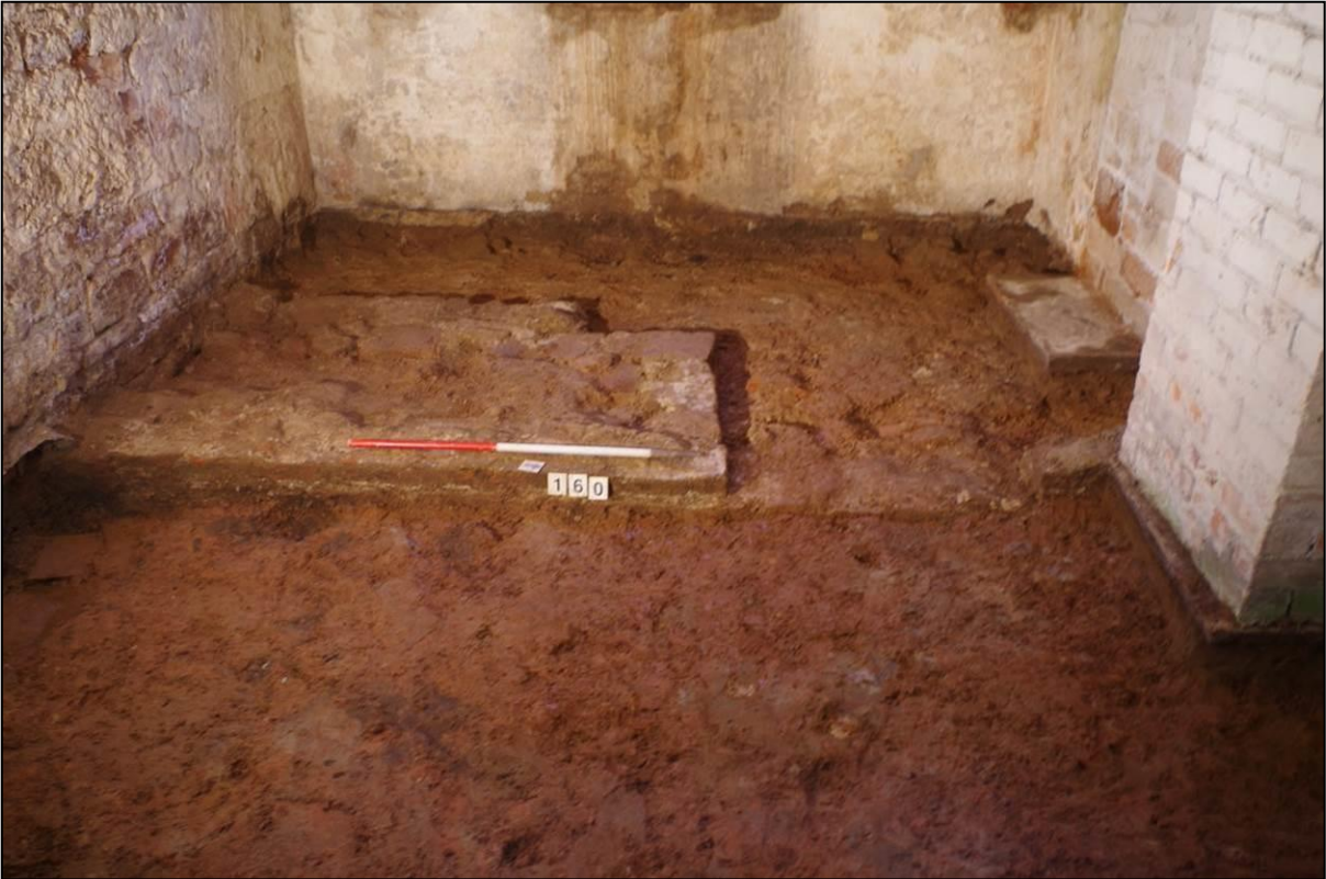
Roman wall within present-day cellar. 58
