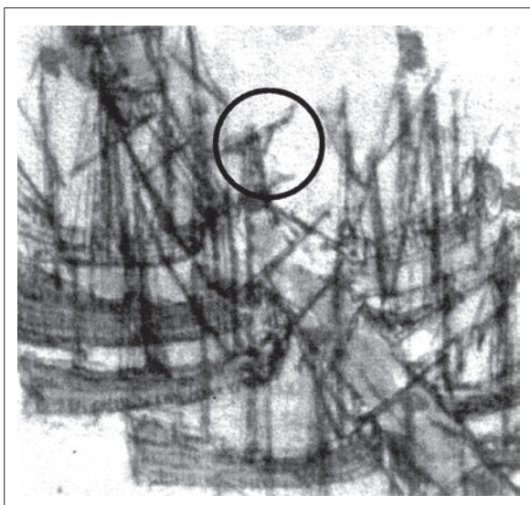
Fig. 16. Jetties at the end of the wooden piers in Stralsund (detail from Stralsunder Staudeplan from 1647).
