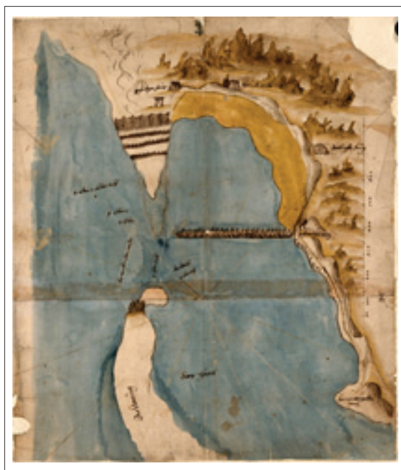
Fig. 13. Wooden constructions were also installed to protect the entrances to harbours, as is seen in an example from Pillau in the 16th century (chart collection of the GSTA Berlin No. 10.803).
