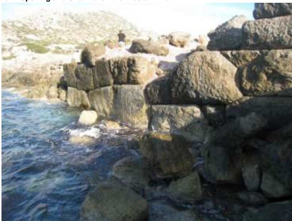
Figure 2: Western Wall of the Breakwater Built with Polygonal Blocks
