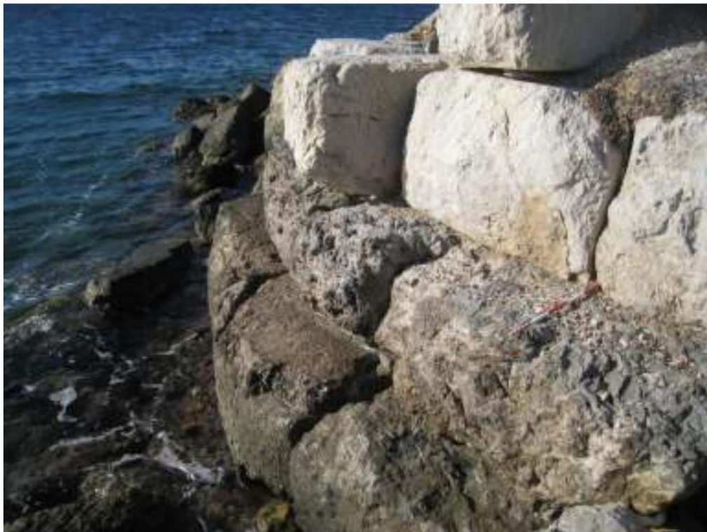
Figure 1: 2-Tier Substructure of Round Tower 2
