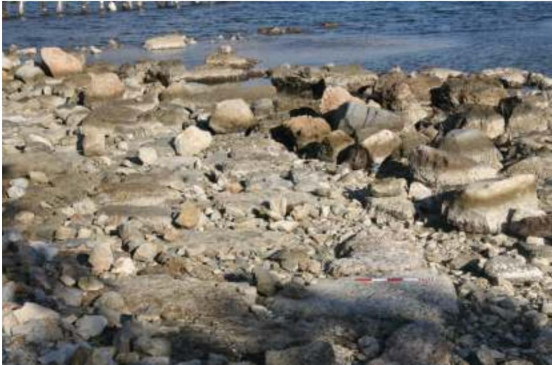
Figure 1: Infrastructure of the Pier Consisting of Conglomerate and Limestone Blocks
