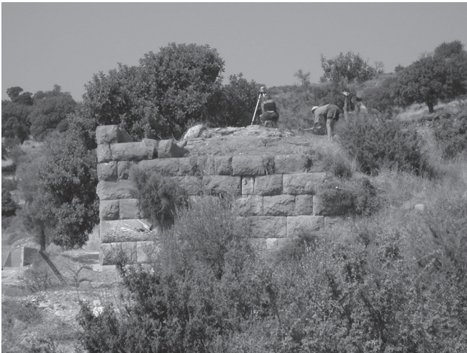
Fig. 19. Tower 10 from the south.
