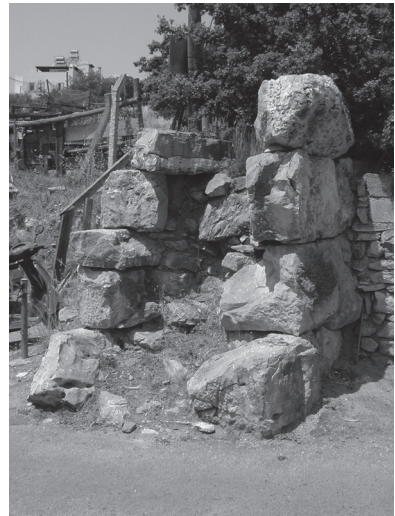
Fig. 38. Southernmost visible part of the east side of the city wall, about 200 meters south of tower 25 .
