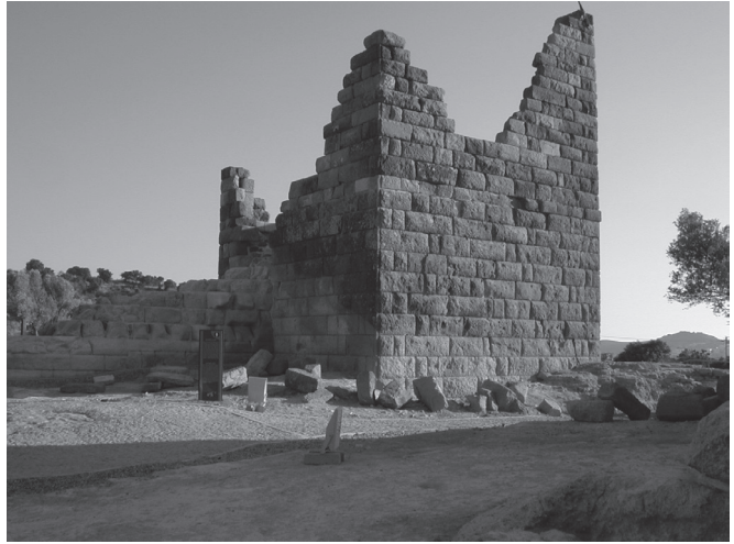
Fig. 13. Myndos Gate. South tower 6 .
