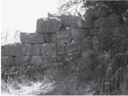
Fig. 5. Irregular polygonal masonry in SW part of the city-wall circuit.
