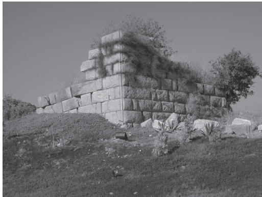
Fig. 6. Tower 4 south of the Myndos Gate.
