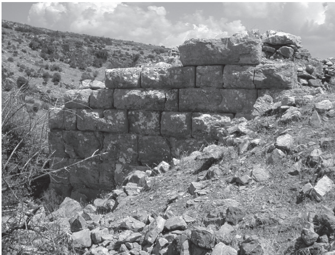
Fig. 31. West side of tower 20 .
