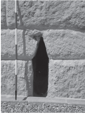
Fig. 12. Myndos Gate. Drainage opening in south side of northern connection-wall.
