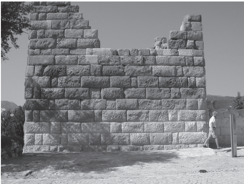
Fig. 45. South side of the southern tower 6 in the Myndos Gate with frequent use of 'double bond' in the corners.
