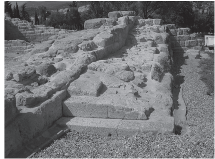
Fig. 10. Myndos Gate. Remains of staircase leading to wall-walk.
