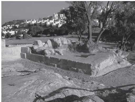
Fig. 7. Tower 5 south of the Myndos Gate.
