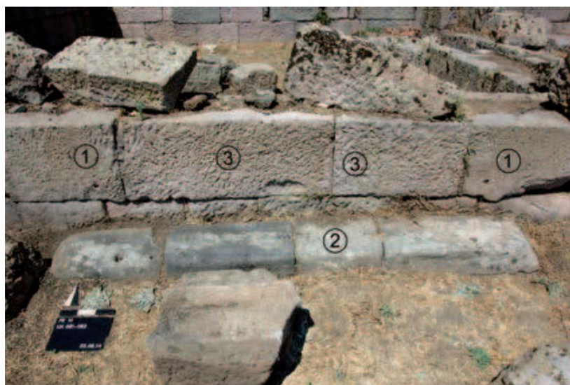
Fig. 52 Pergamon, Stadtberg. Lower agora, room 2. Southern front of the room with original door reveal (1), secondary threshold (2) and subsequent door addition (3)
