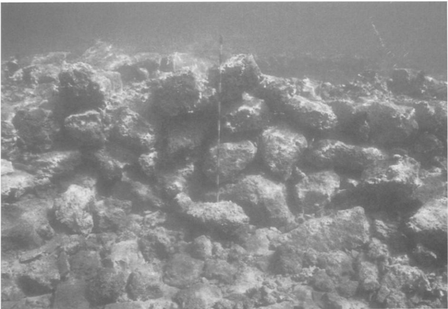
△ Section of Late Antique defensive curtain wall west of jetty, looking north.
