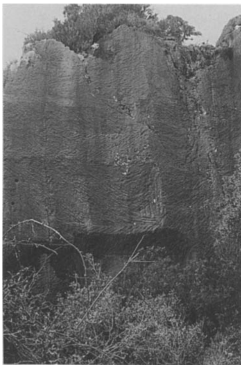
Figure 9. Tool marks: pick with narrow hoop-iron and long wooden handles. Grooves exhibit perpendicular impact on rock. (Photo: authors)
