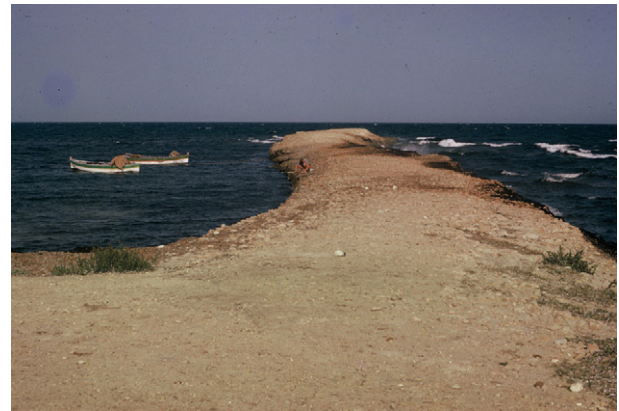
Figure 3. Thapsus Roman 'concrete' mole in 1966, width of mole c.10m. (R. A. Yorke)
