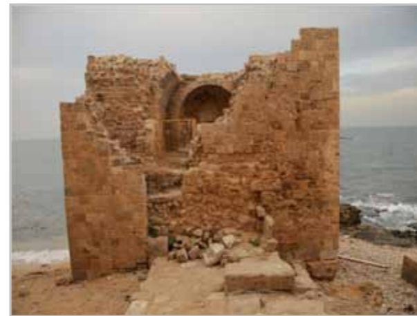
Fig. 12- Al-Moubarkeh Tower located west of Submerged Jetty, looking north.
