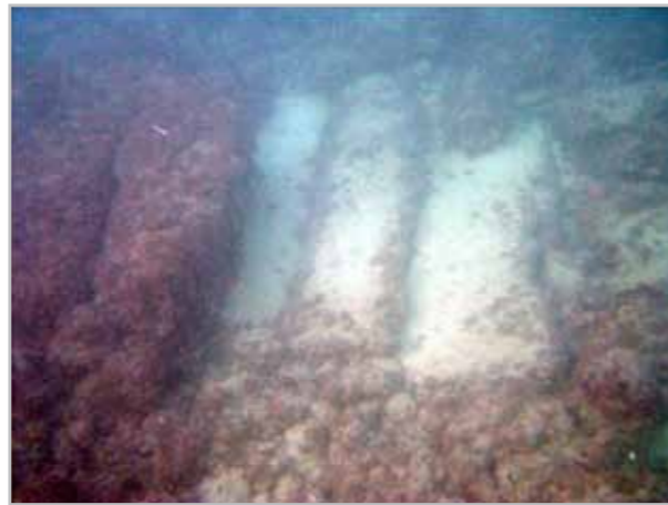
Fig. 14- Evidence of Disturbance Along Upper Course of Historic Jetty, looking north.
