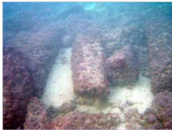
Fig. 15- Additional evidence of Disturbance Along Upper Course of Historic Jetty, looking north.
