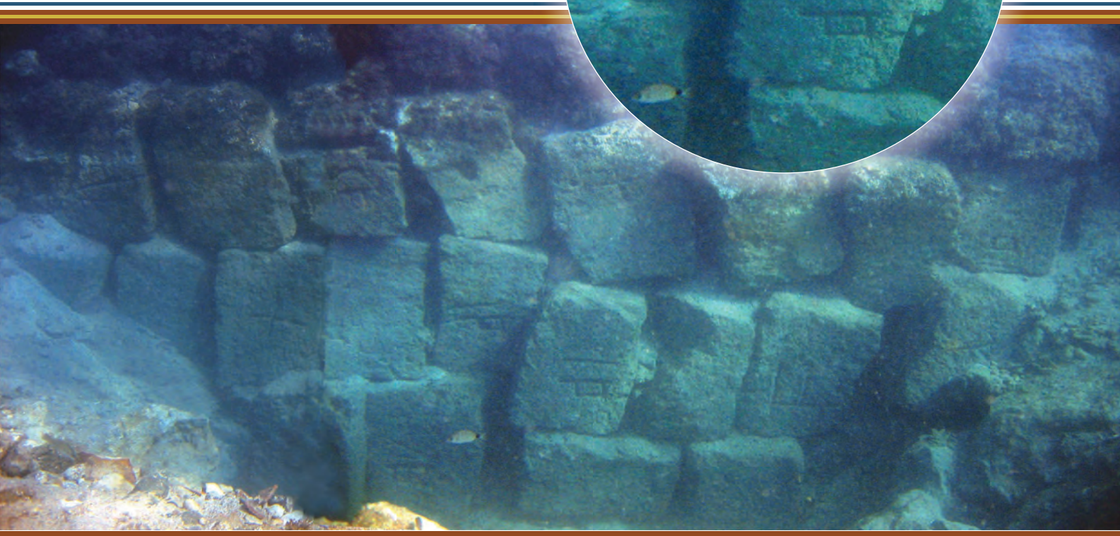
Figure 4. The façade as shown by the sounding test on the inner wall of the jetty. Note the masonry marks on many of the headers (see inset). Photo by Ibrahim Nouredine.
