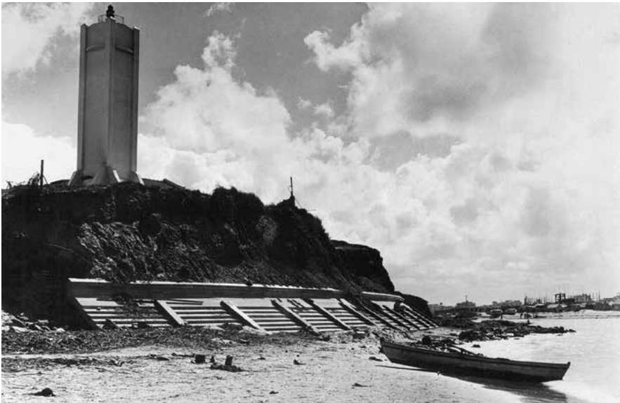
Fig. 22. The lighthouse and the sea wall protecting its foundations at the bottom of the mound cutting the mound western façade (1936/1937), looking south-east (photograph: IEC, historical archive section).
