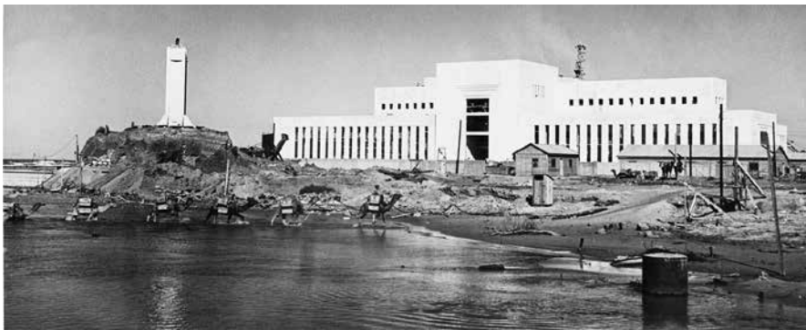
Fig. 32. The mound during excavation, while preparation works were still on the ground and lighthouse base reinforcement took place (the newly built Reading Power Station in the background) (late 1937) (photograph: unknown; IEC, historical archive section).
