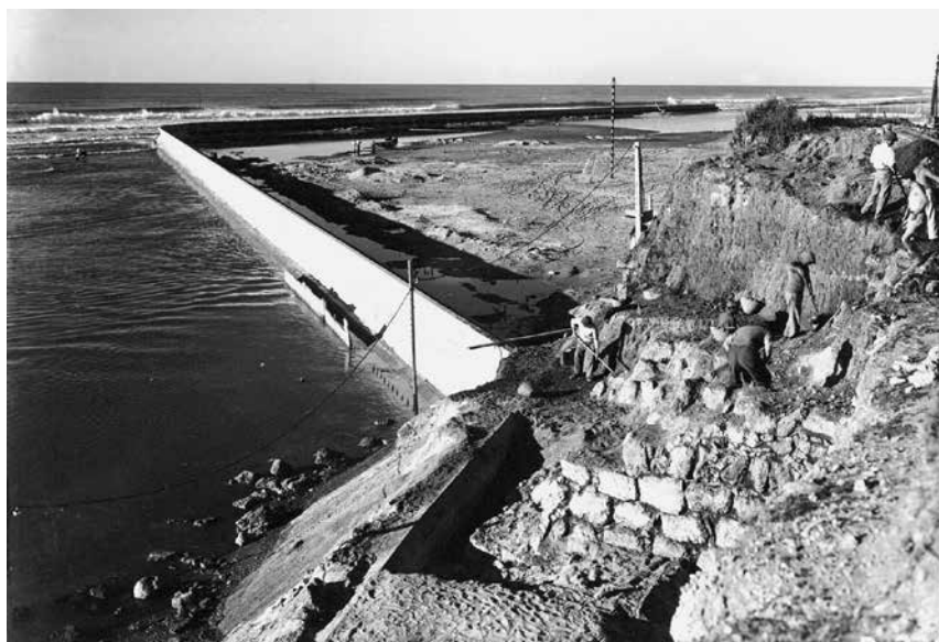
Fig. 29. The mound during excavation and the newly built break water wall of the PEC (Palestine Electricity Corporation) lagoon to its north-west (1937/1938) (photograph: unknown; excavation files).
