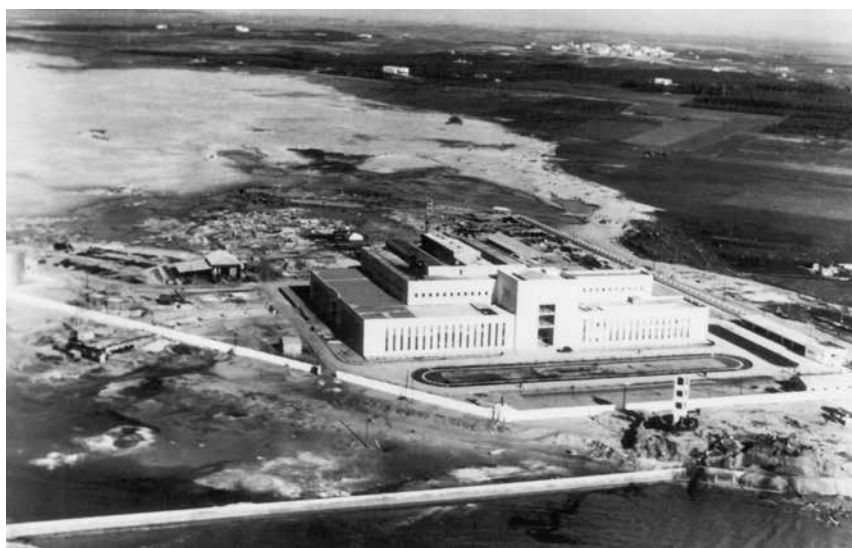
Fig. 30. Aerial photography of the Reading Power Station lagoon during preparation works and its break water wall in the foreground (1938/1939), looking east (photograph: unknown; IEC, historical archive section).
