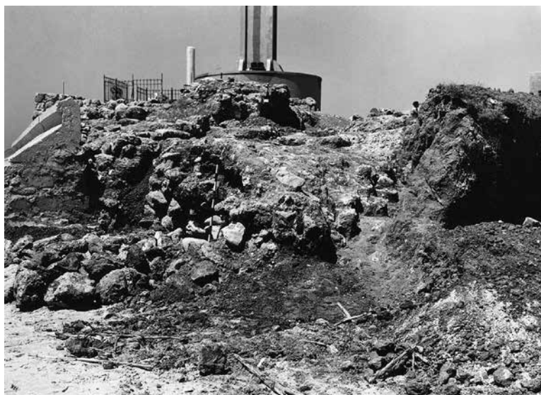
Fig. 34. The lighthouse base after being reinforced (1941), outer rampart wall of the fortress's second stage in the foreground (photograph: unknown; IEC, historical archive section).
