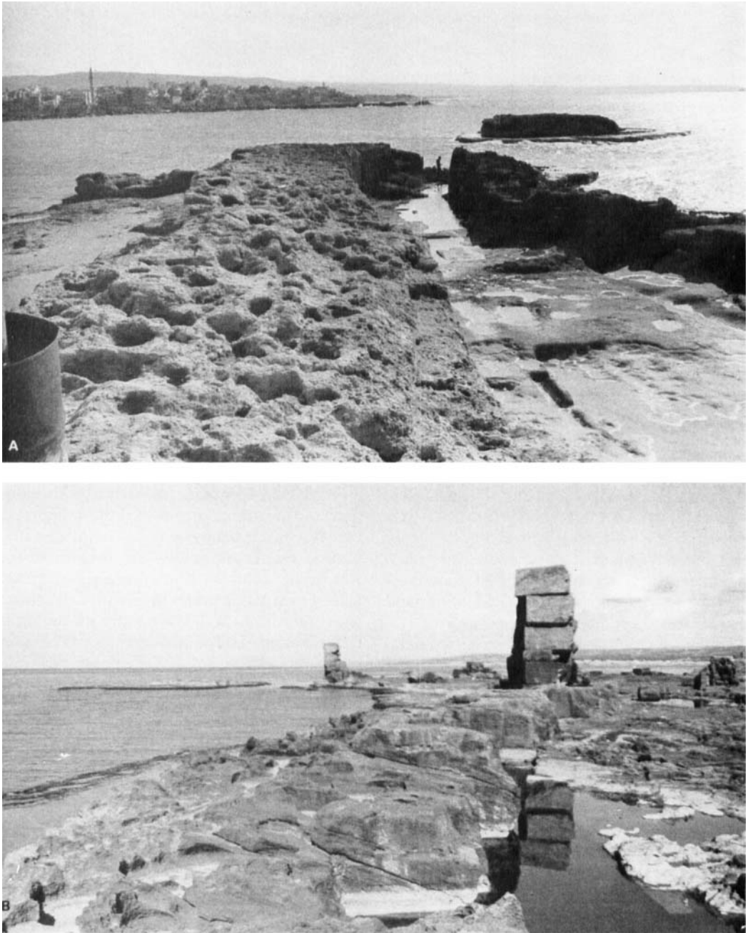
Figure 3. A. Rock-cut sea-walls at Sidon Island (looking towards the Islet); all traces of superstructure have been removed. B. Similar walls on the seaward side of the Island of Arwad; in the middle distance the best-preserved section of the original wall: five courses of blocks set on top of the 2 m-high rock-cut wall (total height 9 m). Another stretch of the original wall can be seen in the background.
