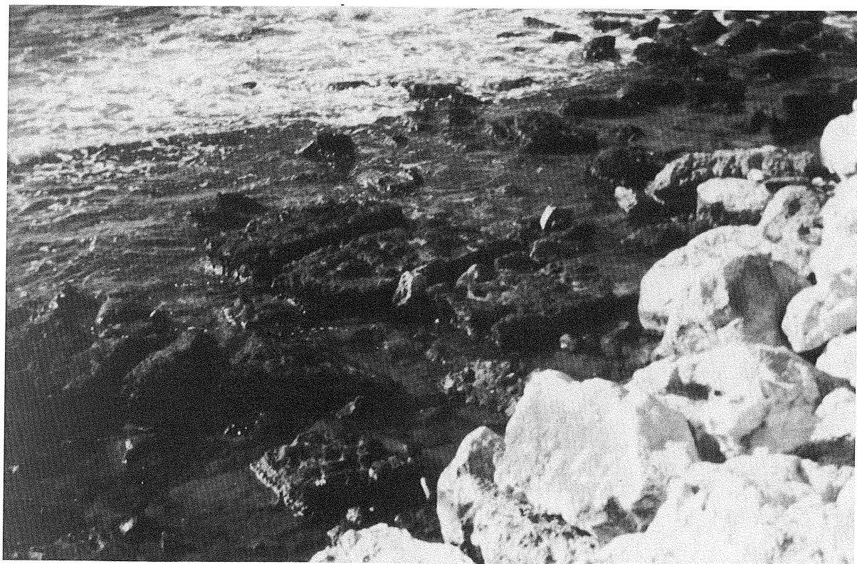
Fig. 37. Ashlar walls of the ancient mole at Marion-Polis, looking to the north.
