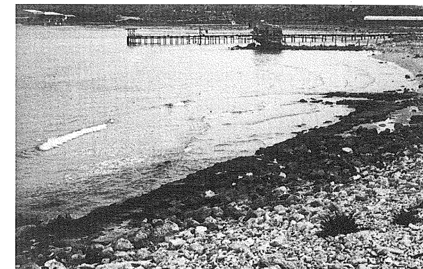
Fig. 25. The southern quay at Athlit and the stem of the double walls of the eastern mole, looking east.
