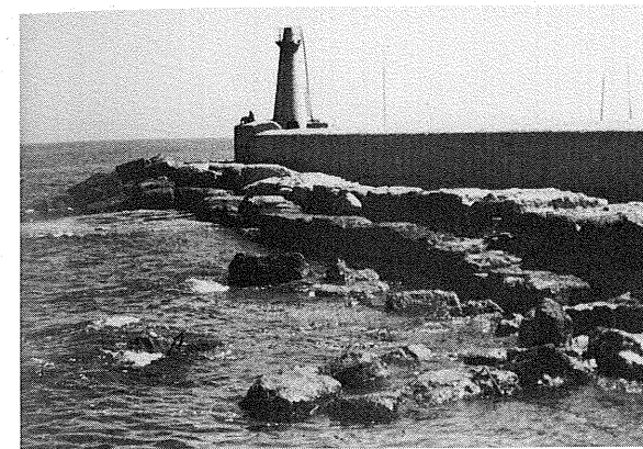
Fig. 40. The ancient ashlars on the western side of the harbour at Kyrenia, of the Roman or Medieval period (?) looking to the NE.
