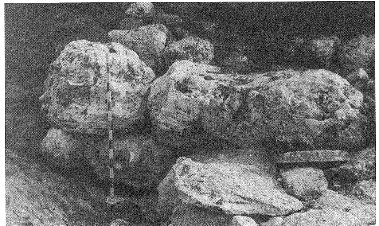
Fig. 7. The MB IIA seawall at "Love Bay" in Dor, looking east.
