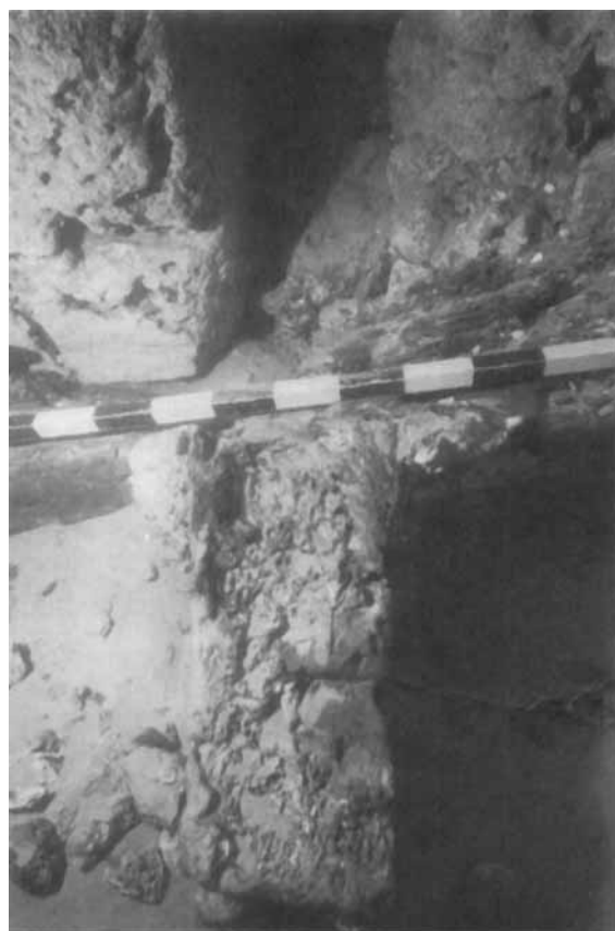
Figure 17. The base beam of the caisson at the corner of two neighbouring blocks.
