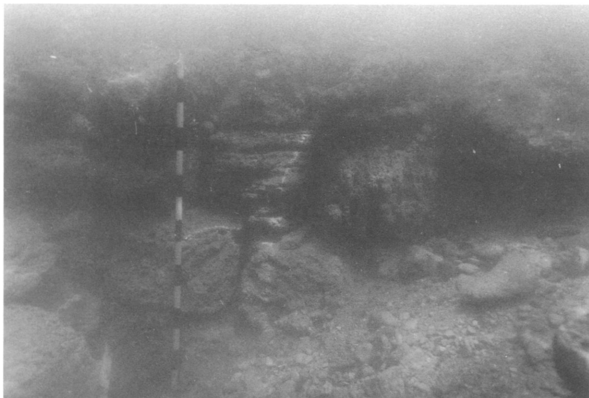
Fig. 5. Submerged courses of headers at the side of the round tower (photo: M. Little).
