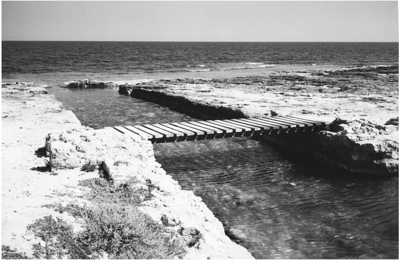
Figure 4.3. The flushing channel at Mahdia, Tunisia (Photograph: A. Raban)
