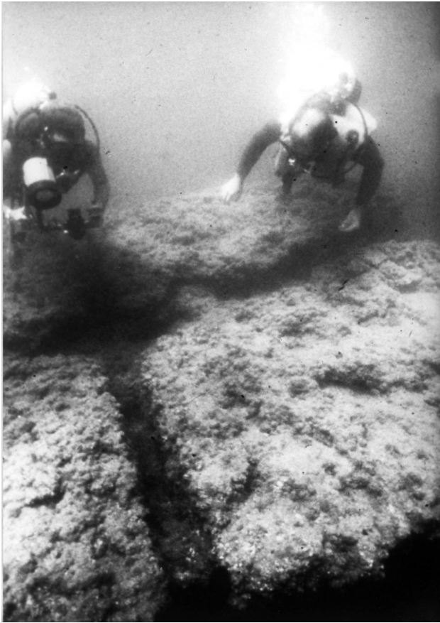
Figure 5.26. The “Negative” grooves of wooden transoms at the surface of one of the segmented blocks of hydraulic concrete at Area C4 (Photograph: A. Raban)
