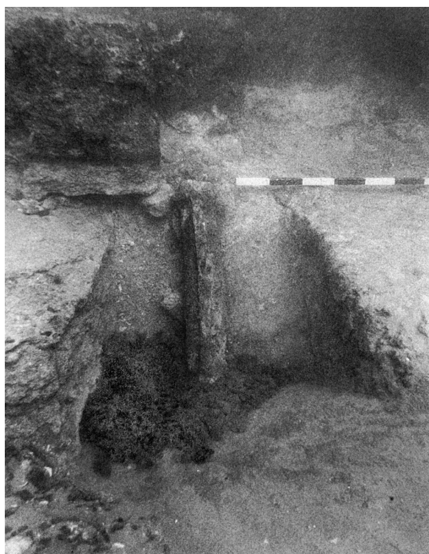
Figure 5.19. Stringer over-rides the floor frames in K2 inner cell (Photograph: A. Raban)
