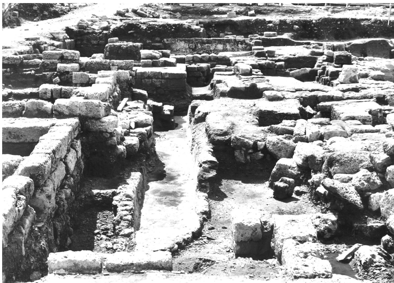
Figure 5.96. The northern-most surviving section of the flushing channel in Area 15, looking southward (Photograph: A. Raban)
