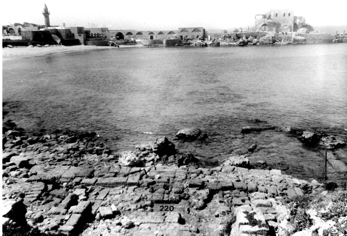
Figure 5.78. The sea wall at Area S, from the north (Photograph: A. Raban)
