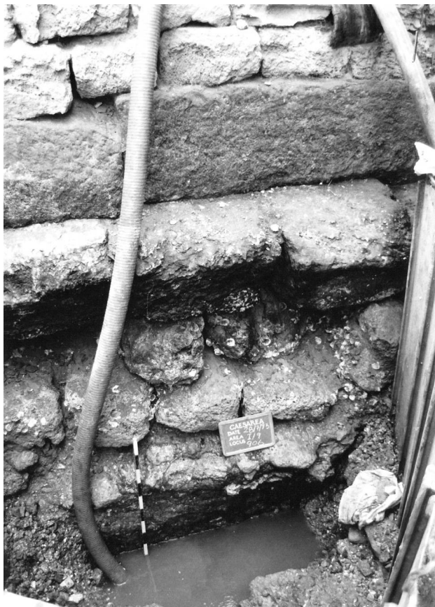
Figure 5.98. The eastern quay at I9, from the west (Photograph: A. Raban)
