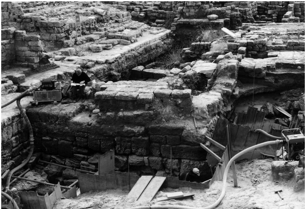
Figure 7.11. A northern elevation of the circular staircase at I-1 (Photograph: A. Raban)
