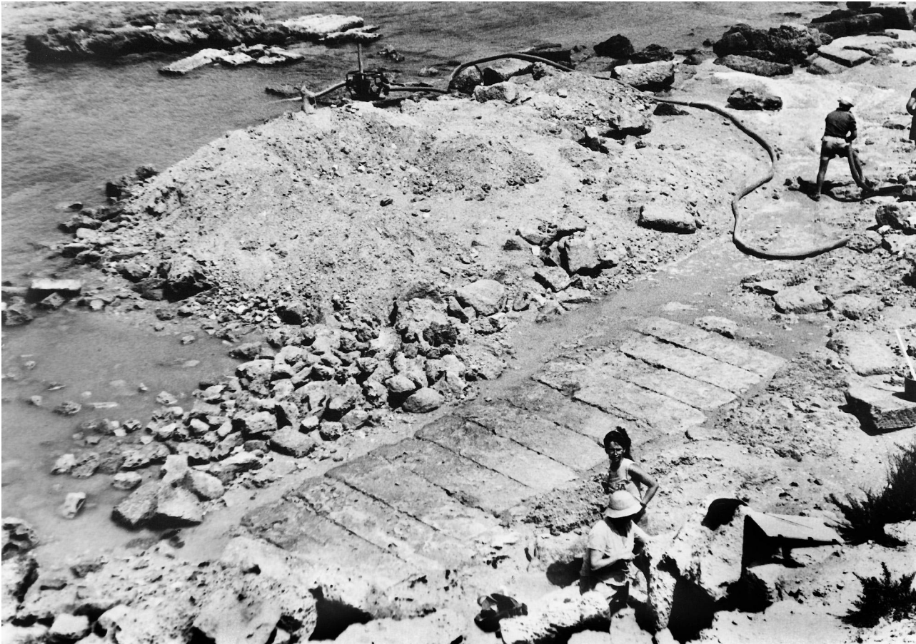
Figure 5.82. The quay at Area L, looking from the south (Photograph: A. Raban)
