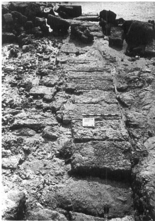
Figure 8. The pier of Area L, looking west. Notice the dovetail grooves at the lower right-hand side (Photo: M. Little).
