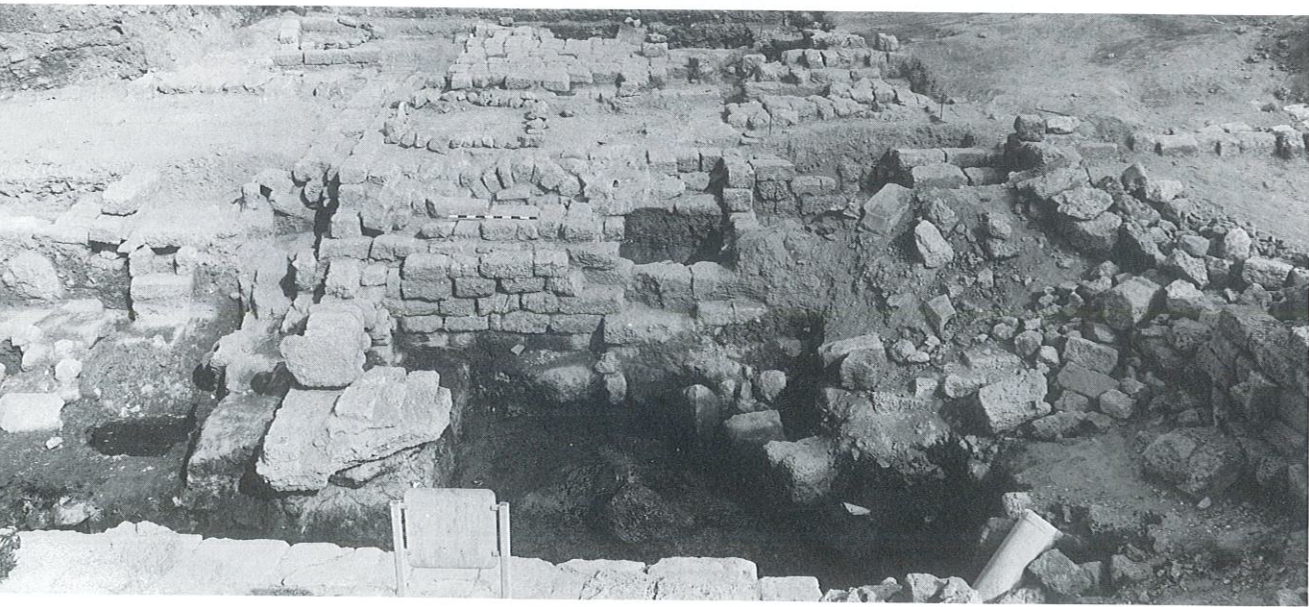
Fig.21. Area I/1, general view to W (1989). In center (just above scale) is vault of a drainage channel 1059, later blocked for use as cistern. In foreground is E quay of inner harbour; just below it is part of a Byzantine reservoir or pool paved with ashlar (ph: Mark Little).
