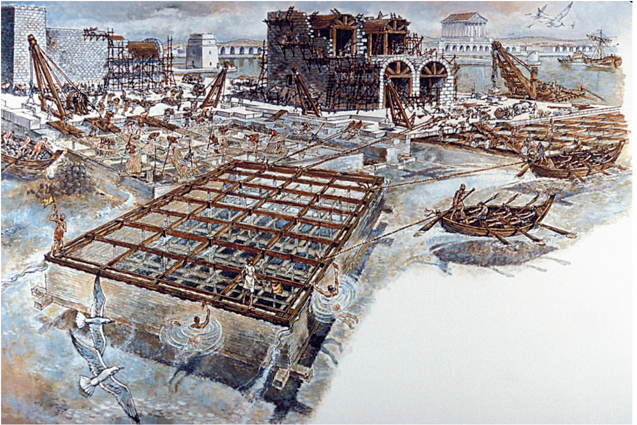
Figure 2.3: Roman marine concrete going into the wooden caisson using trip baskets (painting by Robert Teringo, courtesy of the National Geographic Society, used with permission, after Hohlfelder 1987: 264-265).
