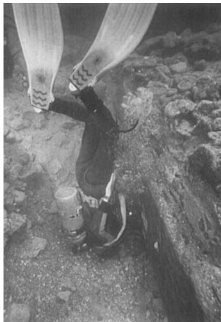
Figure 2. A section of one of the wooden barges at end of North Breakwater. Mortise joints are visible, as is the concrete fill. (Photograph: author).
