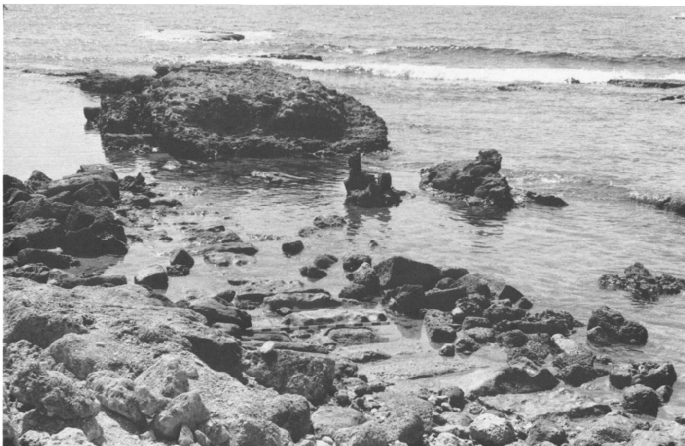
Headers in the foreground mark the Phoenician or Hellenistic quay in the secondary anchorage north of the main facility at Sebastos. The massive rubble structure seaward is part of the Byzantine fortification system probably constructed around A.D. 500. Photograph is by Robert L. Hohlfelder.
