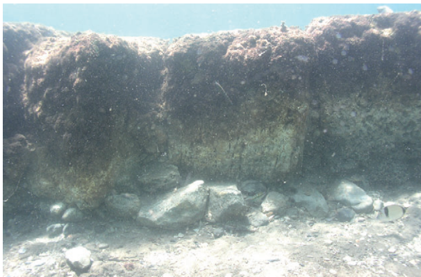
Figure 8. Pebbles placed under the eastern mole foundation for stability. (S. Breitstein)
