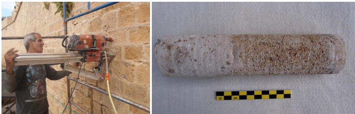
Fig. 7 a, 7b, 7c Drilling of "cores" in the sea walls
