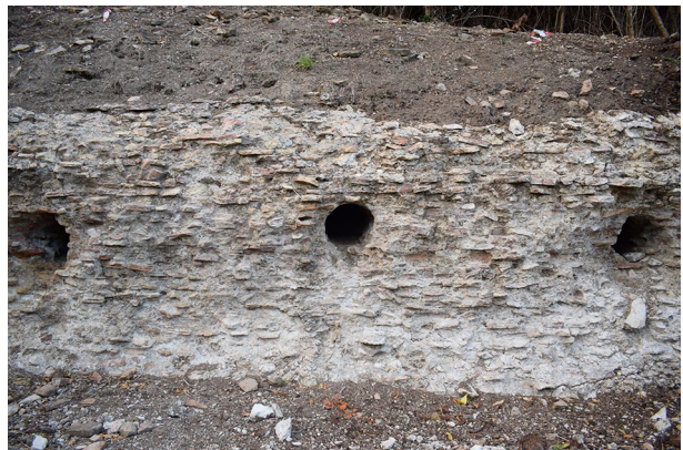
Fig. 7 Detail of the quay wall
