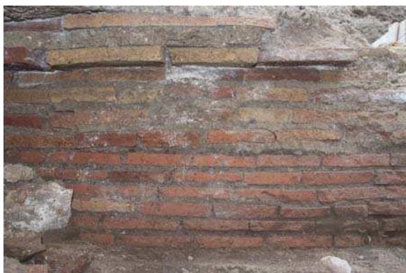
Fig. 17. View of the side of a suspensurae wall with the two construction phases (photo R.A.E. Kok-Merlino).
