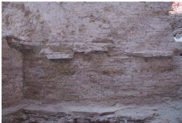
Fig. 14. Wall delimiting the entrance to room B at north-east with traces of the attachment of the floor level and underneath the offset covered with tile fragments, seen from the southwest (photo R.A.E. Kok-Merlino).
