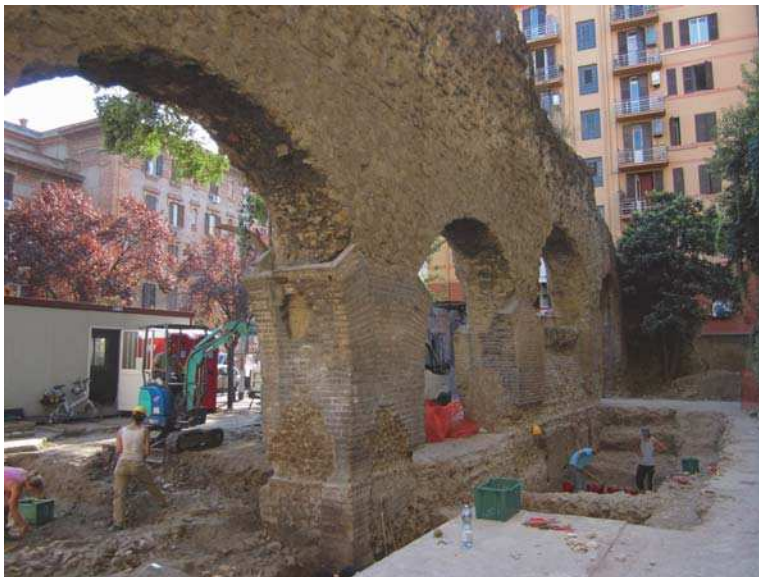
Fig. 1. The excavations in progress (photo C. Tetteroo).
