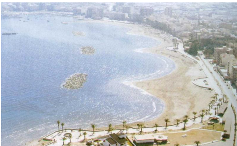
Figure 12.3: Application of offshore breakwaters, Murcia (Spain)
