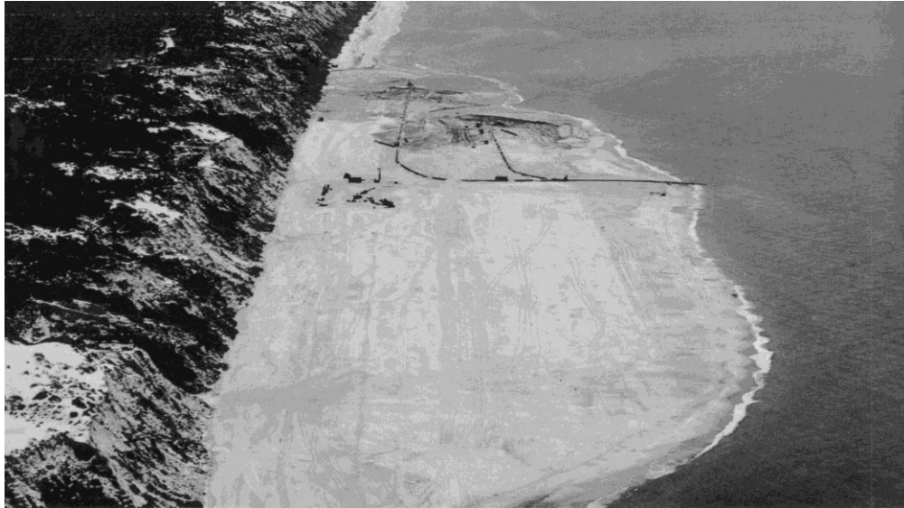
Figure 11.2: Artificial beach nourishment, Castilla (Spain)
