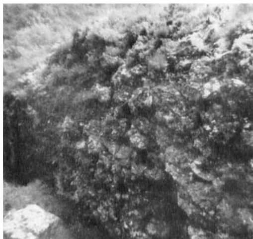
Figure 4. Under water, at depths of 2–10 m, throughout the length of the Cala, there lie great segments of fallen walls made of limestone rubble masonry, like the example shown here.
