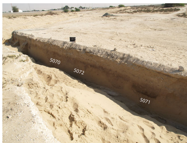
FIGURE 19 Pits (Loci 5070, 5071, and 5072) identified in the main pipeline trench profile indicated in Figure 3 [Colour figure can be viewed at wileyonlinelibrary.com ]
