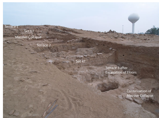
FIGURE 10 The massive post-Wadi Suq collapse found on Terraces 2 and 3 [Colour figure can be viewed at wileyonlinelibrary.com ]
