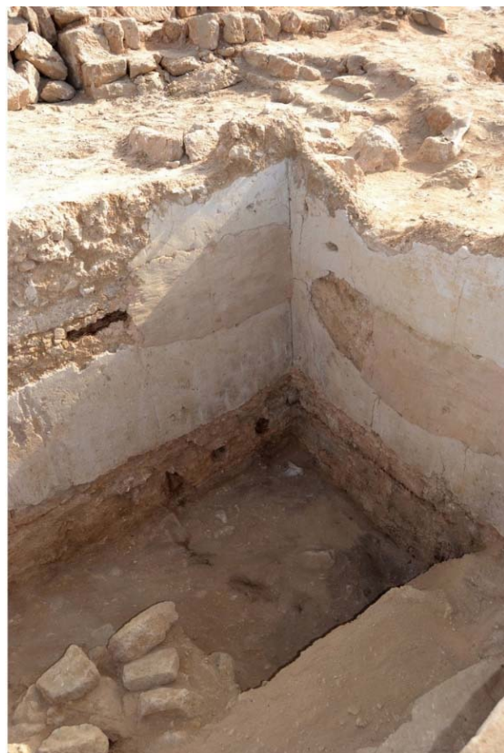
Fig. 36 - Detail of the receiving hall A2 with different layers of plaster on the walls.
