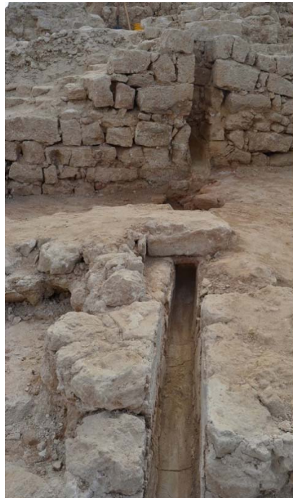
Fig. 40 - Draining channel crossing the western curtain wall.
