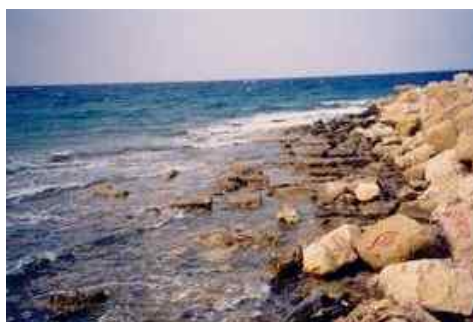
Fig. 5 View of the blocks at the western mole in 2003, before modern reinforcement covered them at all (Theodoulou 1995)
