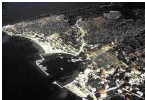
Fig. 3. General view of the two harbours of ancient Thasos as it is today. The submerged mole of the commercial harbour on the upper left corner
