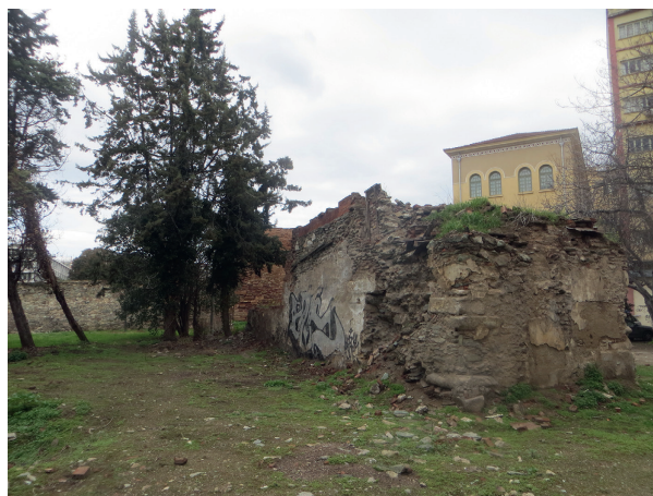
Figure 5.8: Dourgouti Cantilever’s facade from the West (M. Leivadioti).
