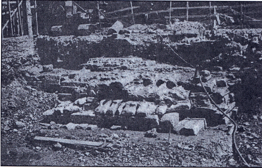
Figure 5.16: The cantilever of the sea wall at 34 Proxenou L. Koromila Street (Bakirtzis 1975: 481, Fig. 2).
