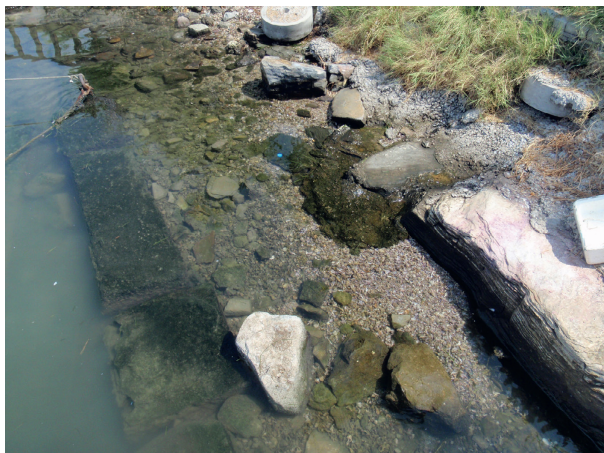
Figure 4.15: A series of flattened blocks and slabs form the walking level of the quay area (A. Ginalis).
