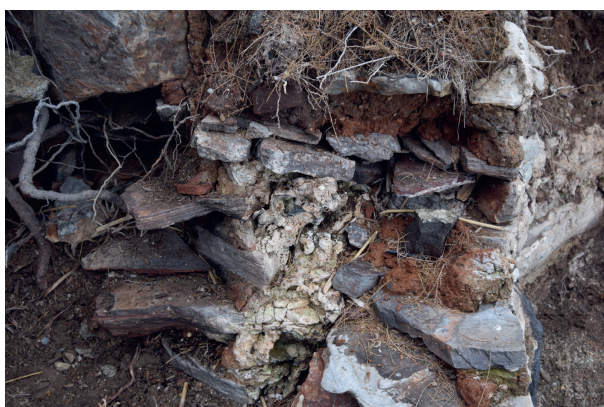
Figure 4.24: Composition of the lower part of the firing chamber (A. Gialouri, Greek Ministry of Culture, Ephorate of Antiquities of Magnesia).
