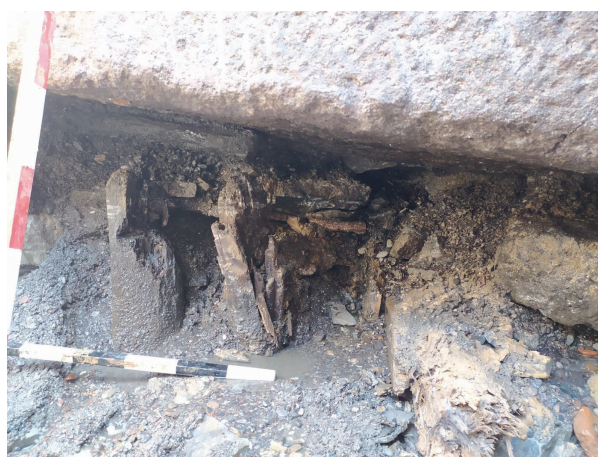
Figure 4.11b: In situ wooden posts of a caisson (A. Gialouri, Greek Ministry of Culture, Ephorate of Antiquities of Magnesia).
