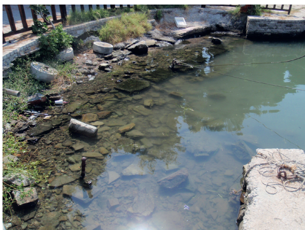
Figure 4.16: Projecting platform from the quay in the harbour basin (A. Ginalis).
