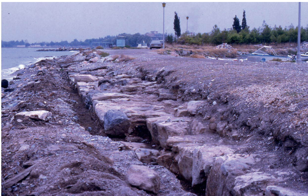
Figure 4.5a: Part of the sea wall along the south-eastern breakwater excavated in 1986 (Greek Ministry of Culture, Ephorate of Antiquities of Magnesia).
