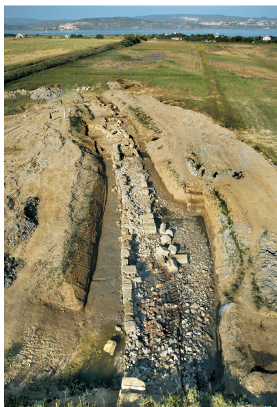
Fig. 1: The wreck used to fill in a breach.
