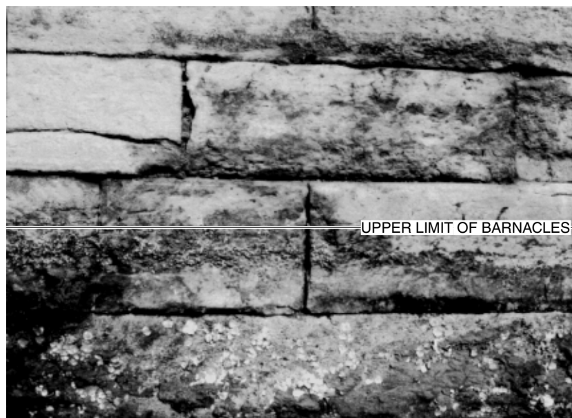
Fig. 5. A well-preserved Roman quay, presenting a continuous upper limit of its barnacle cover. The horizontal limit of the corresponding sublittoral zone is determined by the intact upper limit of barnacles, La Bourse excavation. Photograph: CCJ, MMSH, CNRS.
