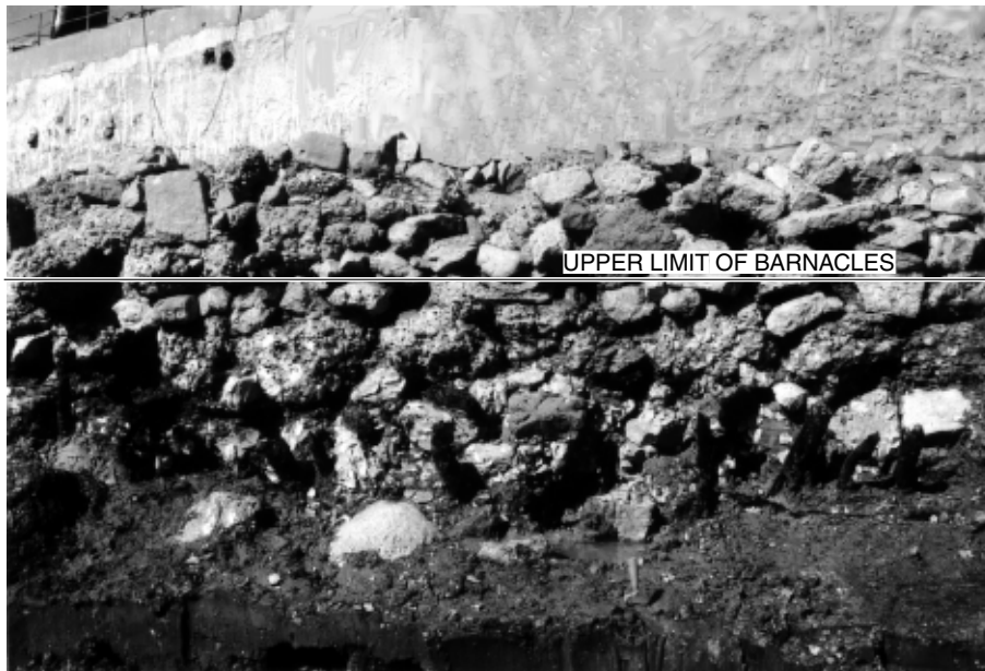
Fig. 3. A well-preserved ancient Greek quay, with contemporary sea floor and presenting an intact and continuous upper limit of its barnacle cover, Villeneuve Bargemon excavation. Photograph: C. Morhange.
