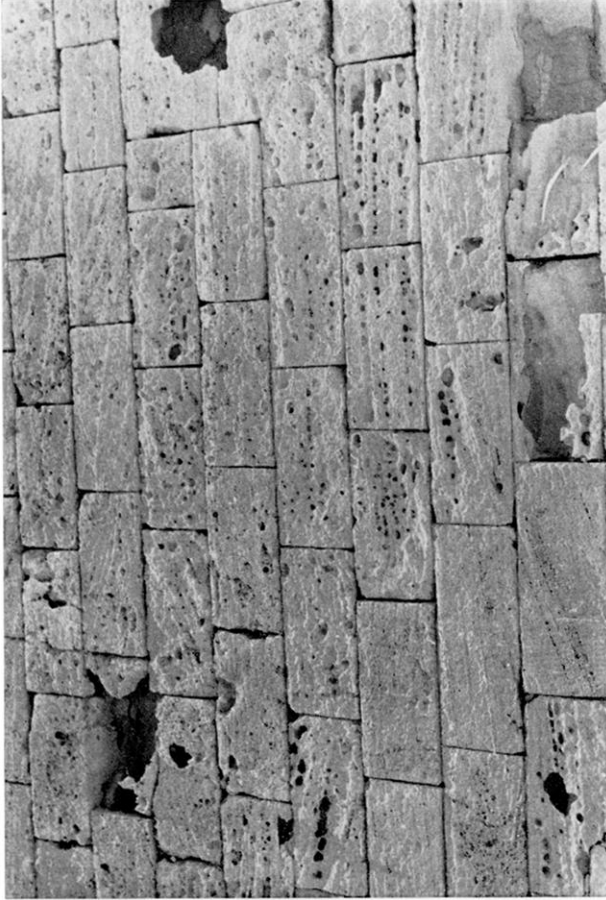
FIG. 6. Temple enclosure, showing Ashlar masonry (smooth surface of blocks).
