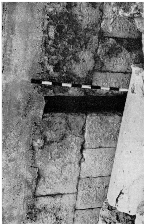
FIG. 8. The Theater of Amman, showing alternate courses of headers and stretchers in the back face of the scaenae frons .
