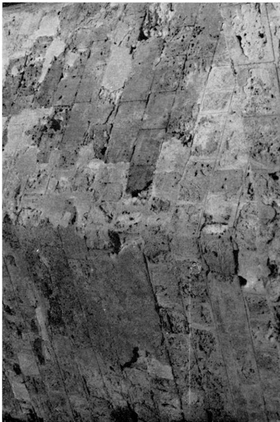
FIG. 7. The Tower, showing alternate courses of headers and stretchers and smooth surface of blocks.
