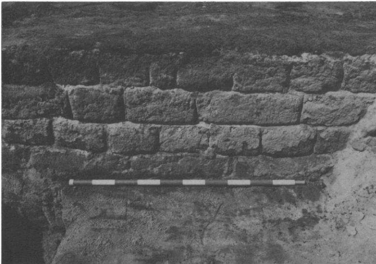
Fig. 6. Section of enclosure wall with layer of burnt deposit on top.
