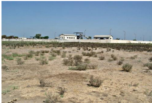
Fig. 43 - Flat area of Kom El-Dahab-II beside the processing plant.
