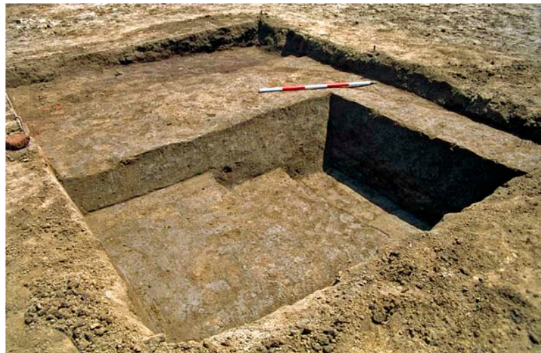
3. Front south-east angle of the temple foundation
