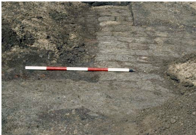
3. Angle of the brick wall and foundation trench in front of the north side of the pylon
