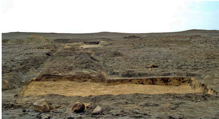
2. View along the pylon foundation from the north
