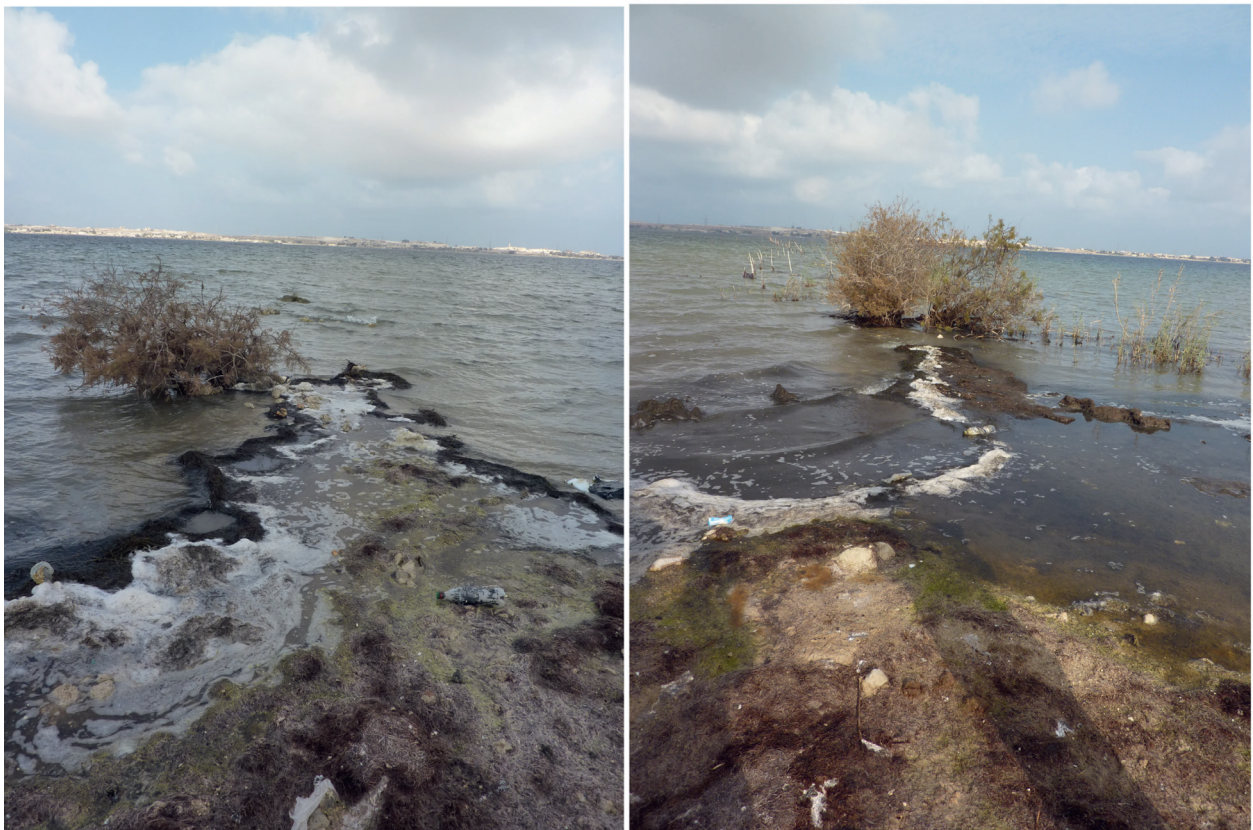
Figure 11.14: Open harbour located between Mariout Island and Philoxenite, Site GMR0056 (based on Google Earth, I. Awad, CEAlex/CNRS).
