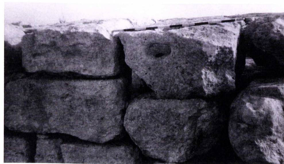
Fig. 2: Kibotos harbour structure, mooring ring (photo M. Haggag).
