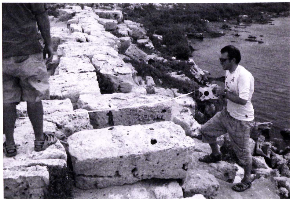
Fig. 5: The quay of Marea harbour was made of large regular limestone blocks without evidence of the use of mortar (photo: E. Khalil).
