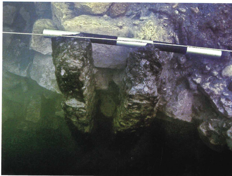
Figure 5.10 Port structures assembled from piles and oak planks ( Quercus sp.), now 3.5 m under water, in the 'Yacht Club' sector of the western part of the Portus Magnus . (Photo: Fernando Pereira © Franck Goddio/Hilti Foundation.)
