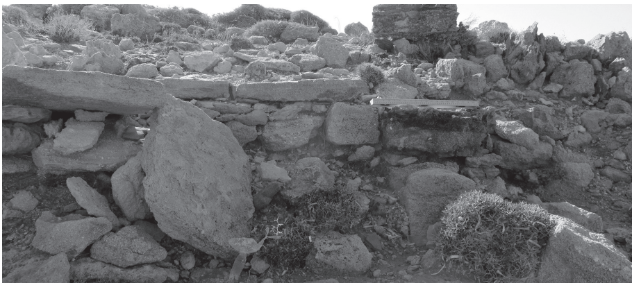
Fig. 8 Detail of the front elevation of the “quay” with flooring slabs (authors).
