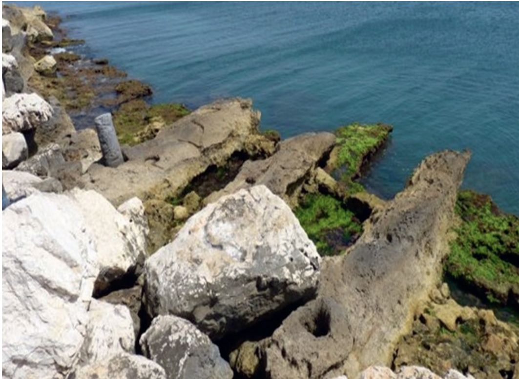
Figure 1.2a: The headers that build the southern mole at the port of Acre (R. Gertwagen).
