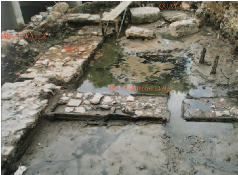
Fig. 16 Harbour structures at Üsküdar. – (Photograph E. Engin, from Karagöz, Khrysolis Liman 413).
