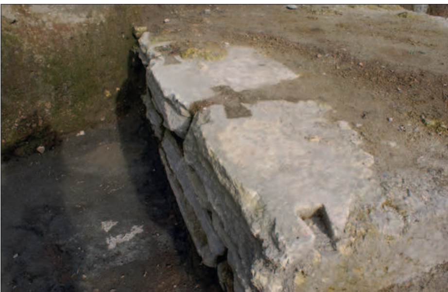
Fig. 12 Yenikapı, grooves for metal clamps at eastern jetty. – (Photograph A. Ercan, from Ercan, Yenikapı 163).
