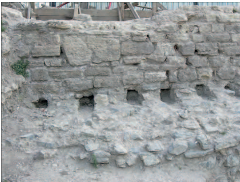
Fig. 32 Yenikapı, row of holes for wooden beams. – (Photograph B. Köşker, IAM Archive, from Gökçay, Architectural Finds 171).
