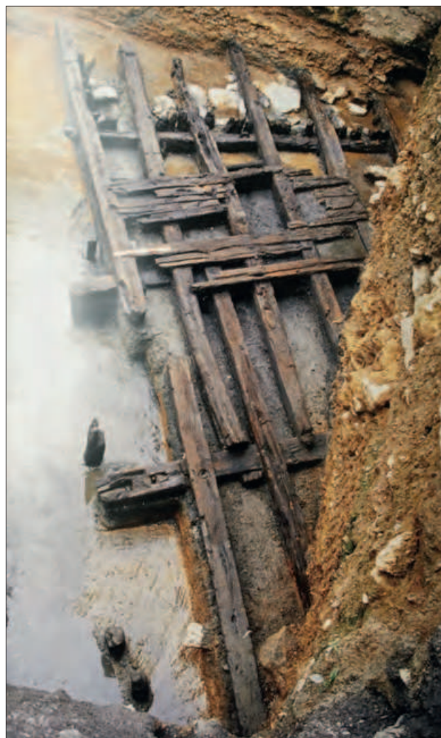
Fig. 54 Wooden pier with cover planks at Üsküdar. – (Photograph Ş. Karagöz, from Karagöz, Marmaray-Üsküdar 104).
