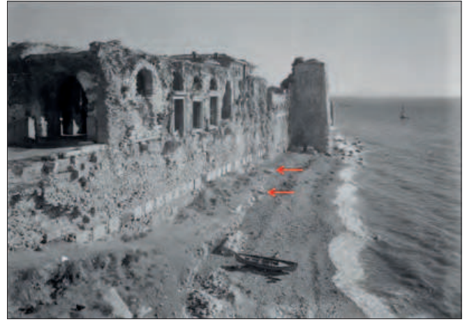
Fig. 48 Chamber system applied at the quayside of the Harbour of the Boukoleon Palace. – (Photograph A. Ginalis after E. Mamboury / Th. Wiegand & G. Berggren, from DAI Istanbul (D-DAI-IST-1020) / http://www.eskiistanbul.net ).
