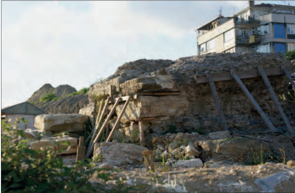
Fig. 21 Yenikapı, western jetty looking north-west. – (Photograph A. Ercan, from Ercan, Yenikapı 162).
