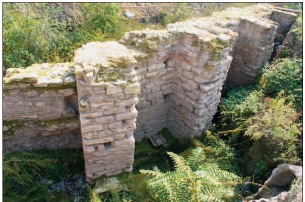
Fig. 34 Yenikapı, part of inner circuit wall enclosing the harbour basin. – (Photograph A. Ercan, from Ercan, Yenikapı 159).
