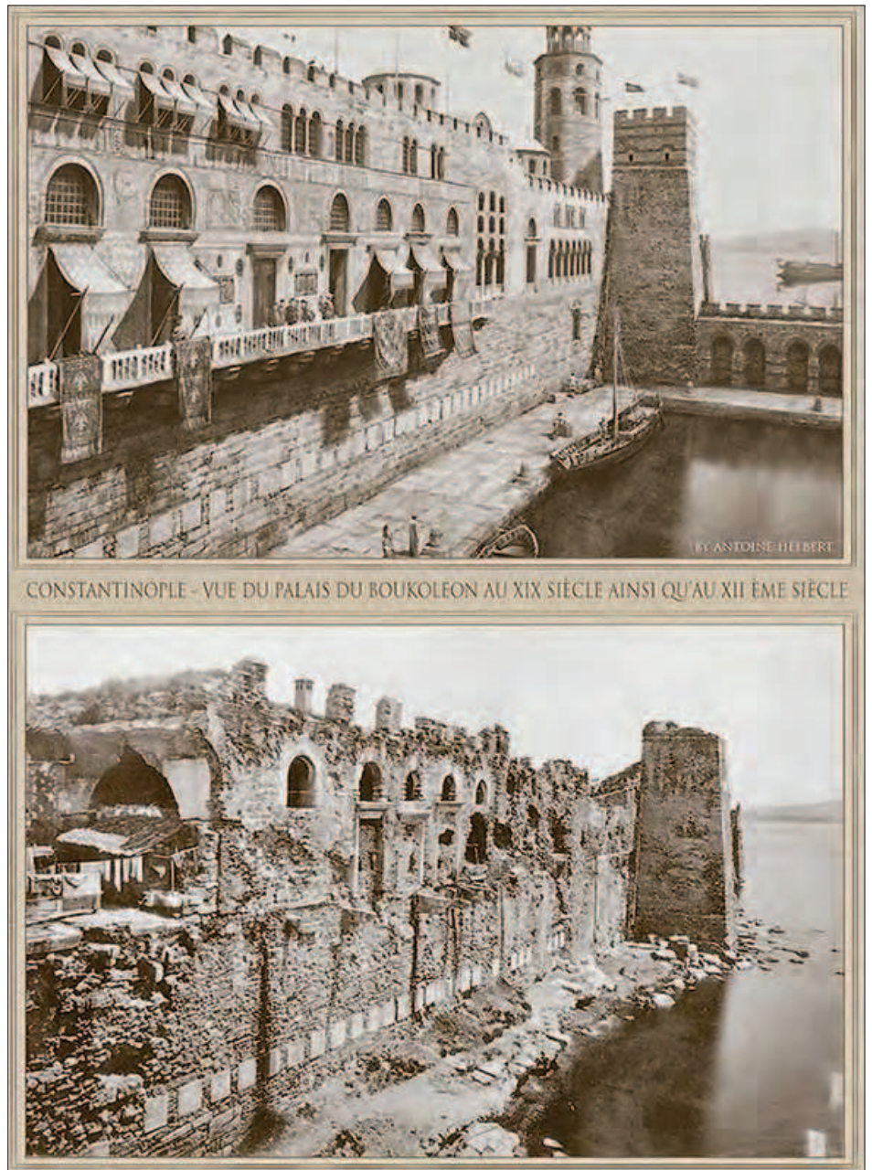
Fig. 48 Chamber system applied at the quayside of the Harbour of the Boukoleon Palace. – (Photograph A. Ginalis after E. Mamboury / Th. Wiegand & G. Berggren, from DAI Istanbul (D-DAI-IST-1020) / http://www.eskiistanbul.net ).
