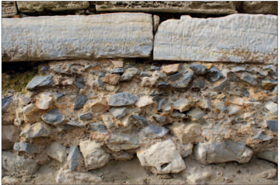
Fig. 7 Yenikapı, concrete filling of the wooden formwork. – (Photograph A. Ercan, from Ercan, Yenikapı 122, detail).
