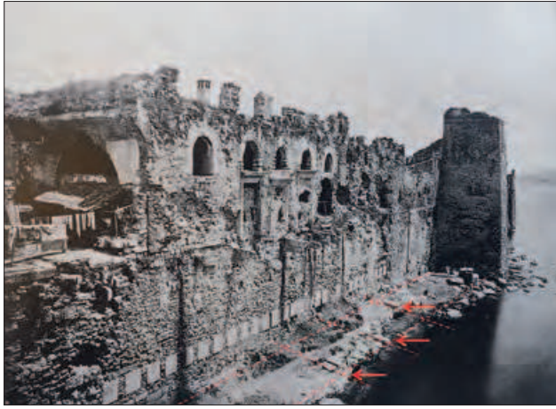
Fig. 48 Chamber system applied at the quayside of the Harbour of the Boukoleon Palace. – (Photograph A. Ginalis after E. Mamboury / Th. Wiegand & G. Berggren, from DAI Istanbul (D-DAI-IST-1020) / http://www.eskiistanbul.net ).
