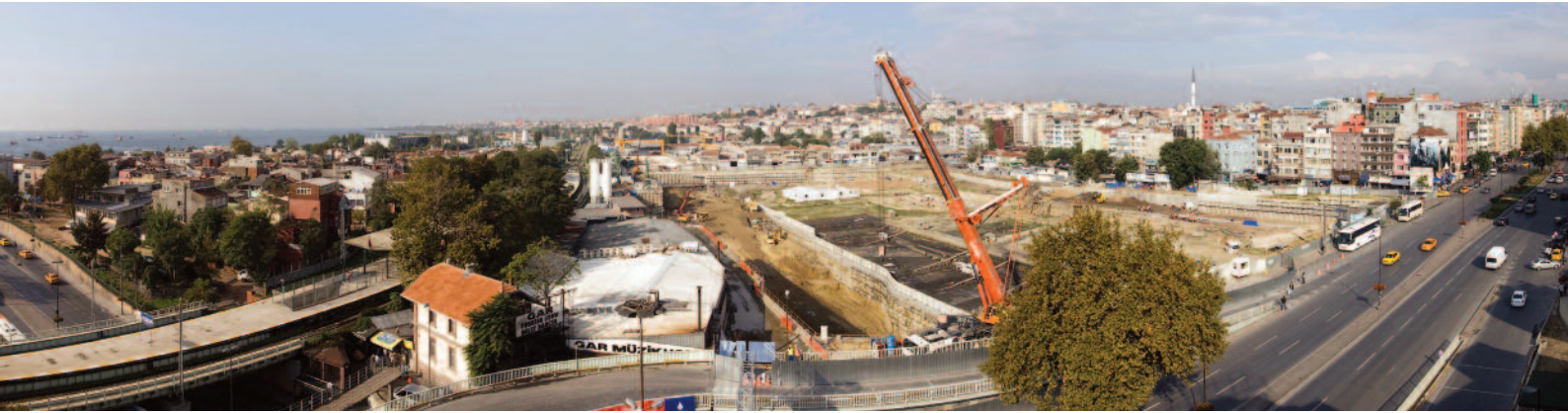
Fig. 3: Yenikapi District and Marmaray-Metro Salvage Excavations.
