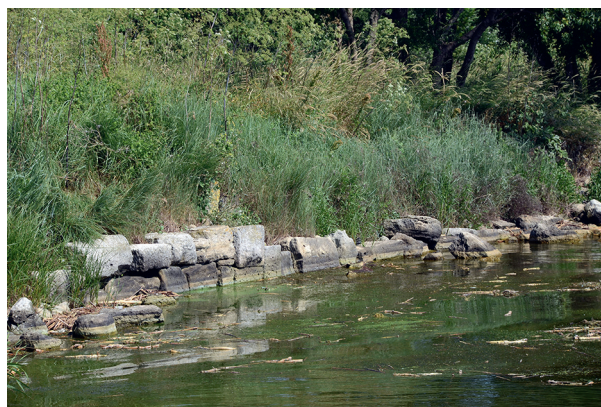
Figure 8.3a: Bank reinforcement (Bathonea Excavation Archive).
