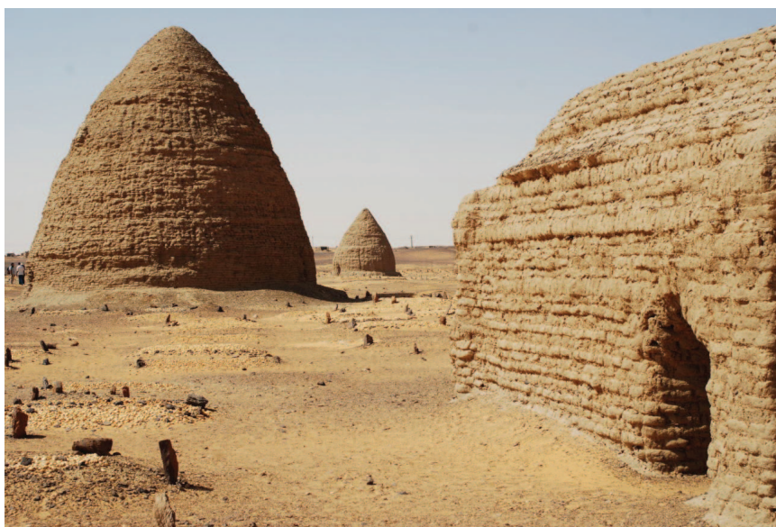
Figure 2. Mud-brick qubba in the cemetery from the Islamic period near Dongola, Sudan. Qubbas are domed mausoleums which contain the grave of a saint or some important personage.
