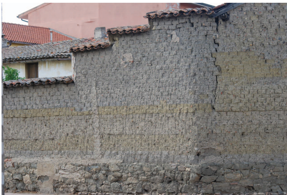
Figure 6. Mud-brick walls in Sardinian houses. Traditional earthen architecture is preserved alongside to modern concrete building.
