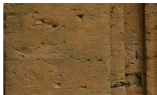
Fig. 4 The thin mortar joints masonry in prospect.
