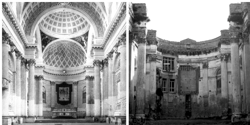
Fig. 1 The church before the roof demolition (left) and in 2002 (right).
