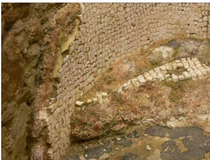
Fig. 1 joint mortar of the internal mosaic lining of the tank at the monumental door
