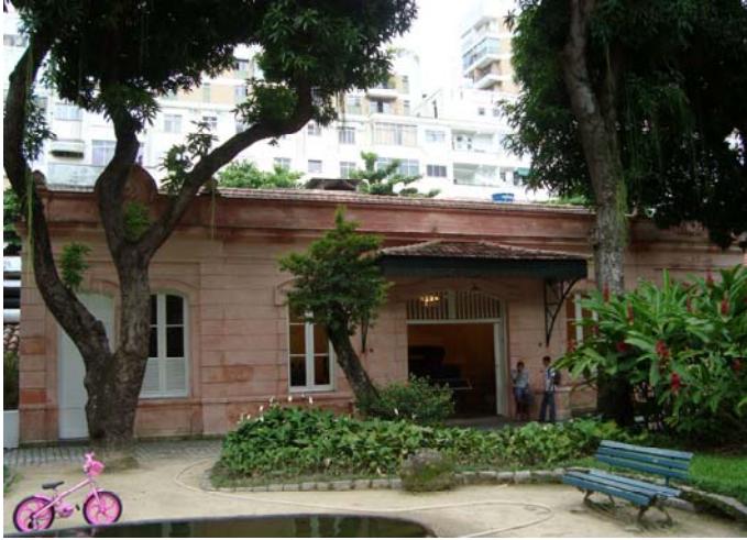
Fig. 4 Stable façade restored with lime plaster two years after the intervention.
