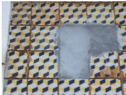
Fig. 6 Filling in of space left by tiles with a cement mortar
