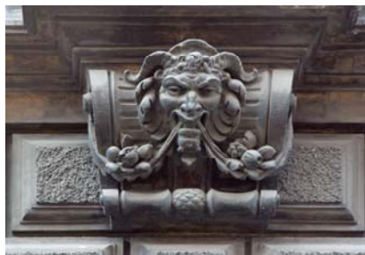
Fig. 2 Original cast decoration and rusticated ashlar blocks: private house, Vienna
