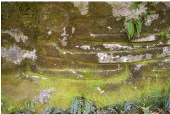
Fig. 1 Detail of a permanently water saturated ignimbrite wall containing carved canoes. The water flow and plant roots are causing delamination in many places.
