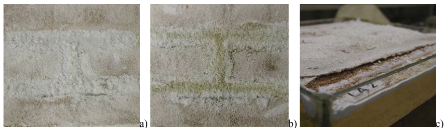
Fig. 3 Distribution of efflorescences on different wallettes during the first cycles
