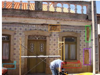
Fig. 7 Sampling of tiles from façade – sampling areas
