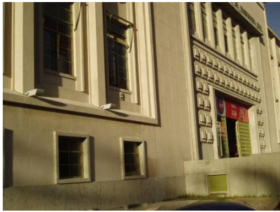
Fig. 13 Main LNEC building: repair with air lime mortar
