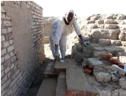
Fig. 5 Applying lime render to brick capping
