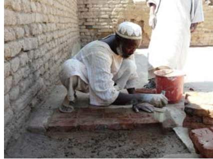
Fig. 4 Pointing the bedded bricks
