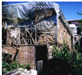
Fig. 2 The storehouse under restoration
