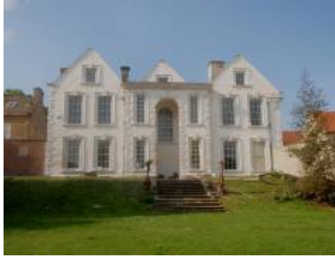
Fig. 3 S elevation, York House, Malton. Central range and windows introduced around 1690, using earth and 5% quicklime mortars and hay-rich earth plasters with limestone dust, quicklime and oxhair finish coats over.
