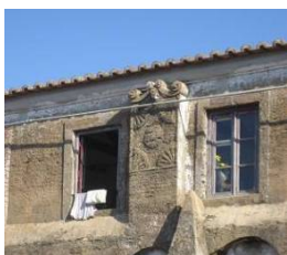
Fig. 5 Relief mortar works
