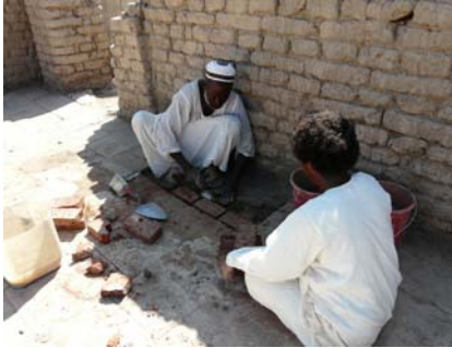
Fig. 3 Laying bricks in a missing area of floor
