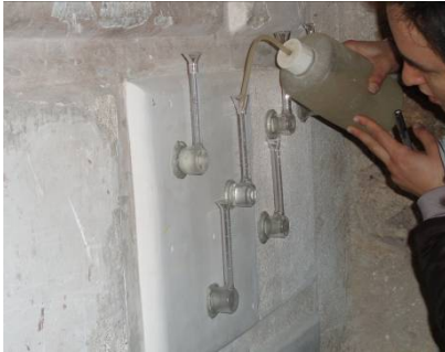
Fig. 9 Evaluation of water permeability with Karsten tubes
