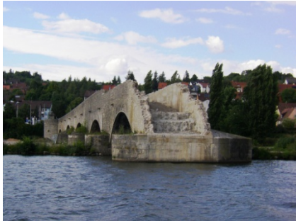
Fig. 1 Northern vaults of the bridge
