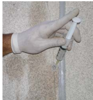
Fig. 6 Repair of render detachment using grouts is a delicate, complex technique
