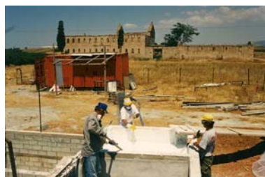
Fig. 7 Wet slaking at the worksite, 2001
