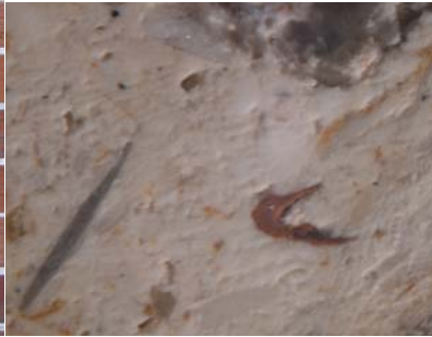
Fig. 4 Mortar in cross section
