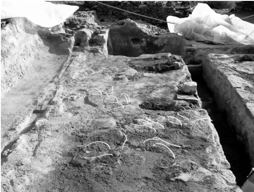
Fig. 2. Washery working floor with remnants of plaster and tailings during grouting
