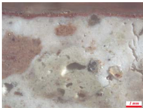
Fig. 3 Polished cross section in reflect light of the crushed brick mortar with a red painted layer coming from the external wall of the octagonal hall
