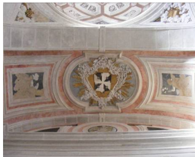
Fig. 17 Stuccoes after restoration.
