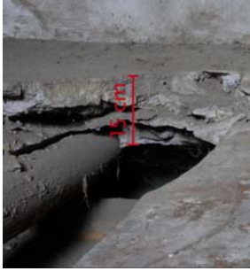
Fig. 3 Ceiling constructions in room 5
