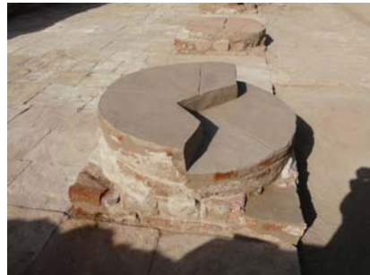
Fig. 6 Finished lime render on column
