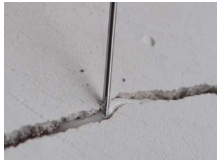
Fig. 8 Filling of cracks with the developed injection grout
