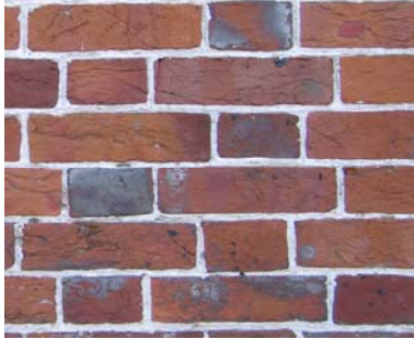
Fig. 3 Mortar joint in situ
