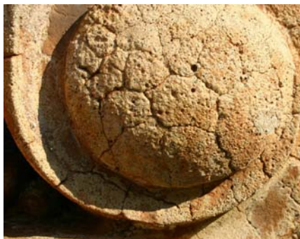
Fig. 2 Heavily eroded surface of a decorative element exposed to rain water; the shrinkage cracks are widened.
