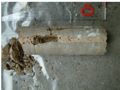
Fig. 3 Drill core with various mortar types
