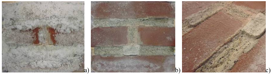
Fig. 4 Surface of MA wallette after 4 weekly cycles: before (a) and after (b) brushing (c) detail of MA wallette after 4 weekly cycles: severe scaling of the mortar can be observed.
