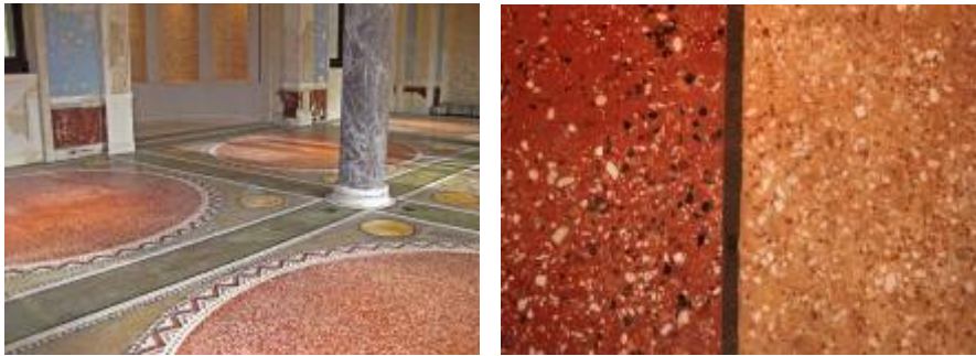
Fig. 12 New Museum in Berlin: Overview and detail of the terrazzo floors made using high fired gypsum as a binder material (photos: Kaiser)
