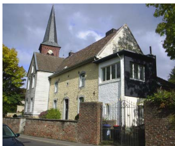
Fig. 3 Rectory of St. Peter in Aachen - gable before the conservation
