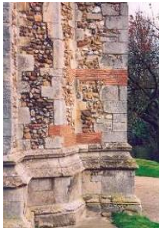
Fig. 3 Honest repair in plain clay tiles to limestone and flint substrate
