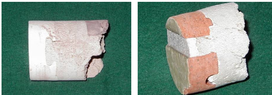
Fig. 3 Two drilling cores from the facades. On the left a drilling core with tiles that are coloured in the mass, on the right a core from a façade with tiles with a superficial colouring. Note the mechanical ‘hooks’ on the back of the tile (left photo) that ensure a good mechanical adherence. Also note structure of the façade on the left photo, with from right to left the structural masonry (a part of a brick is visible), the bedding mortar, the tile. On the right photo also the pointing mortar between the two tiles is visible.
