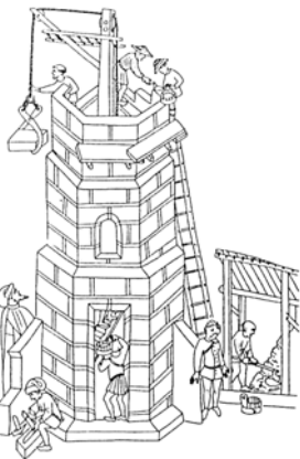
Fig. 3 Mortar prepared in an open hut
