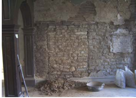
Fig. 4 York House interior, mud-mortared limestone to original wall and late 17thC blocking of original doorway.
