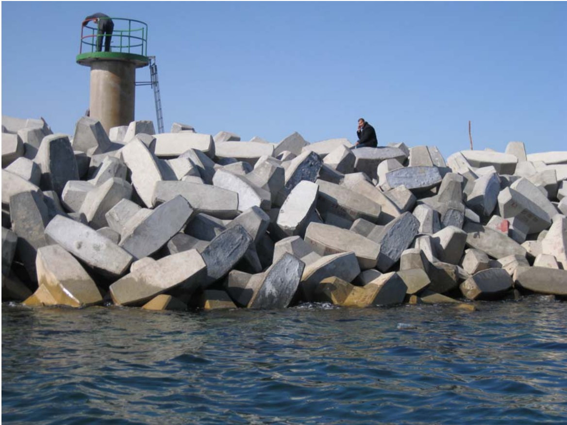
Photo no. 7 – Digue Nord
