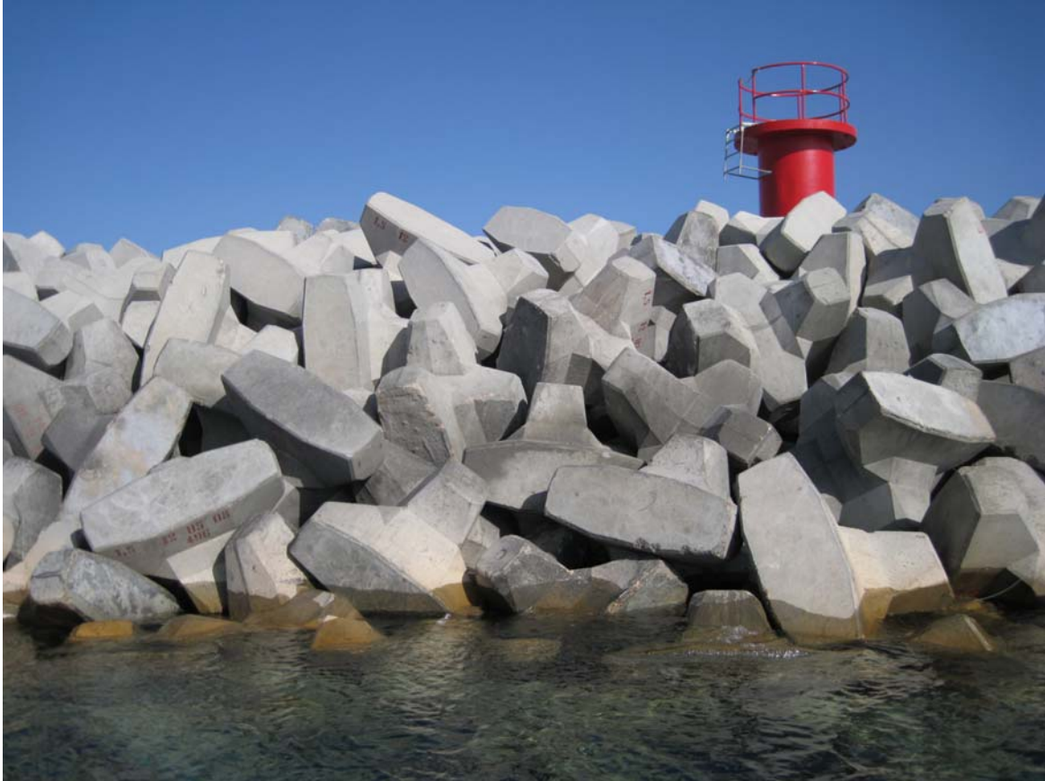
Photo no. 5 – Digue Sud - Musoir
