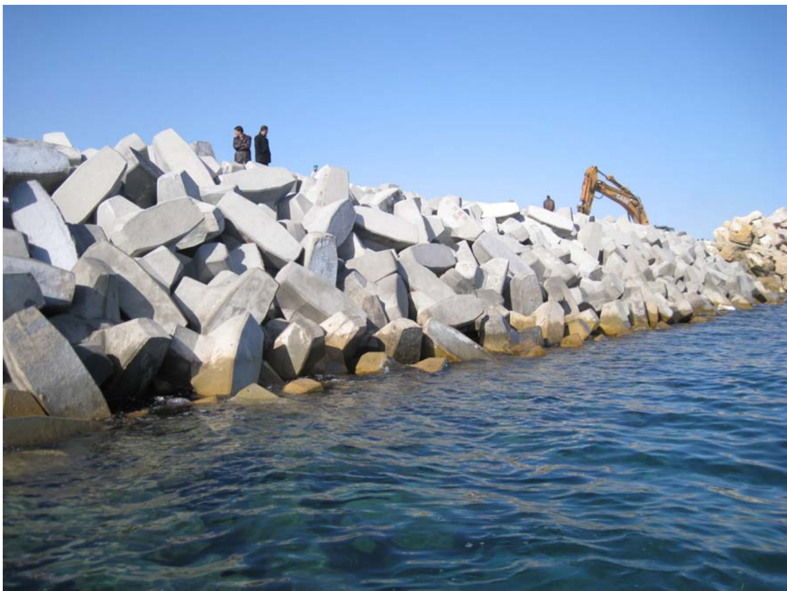
Photo no. 8- Digue Nord
