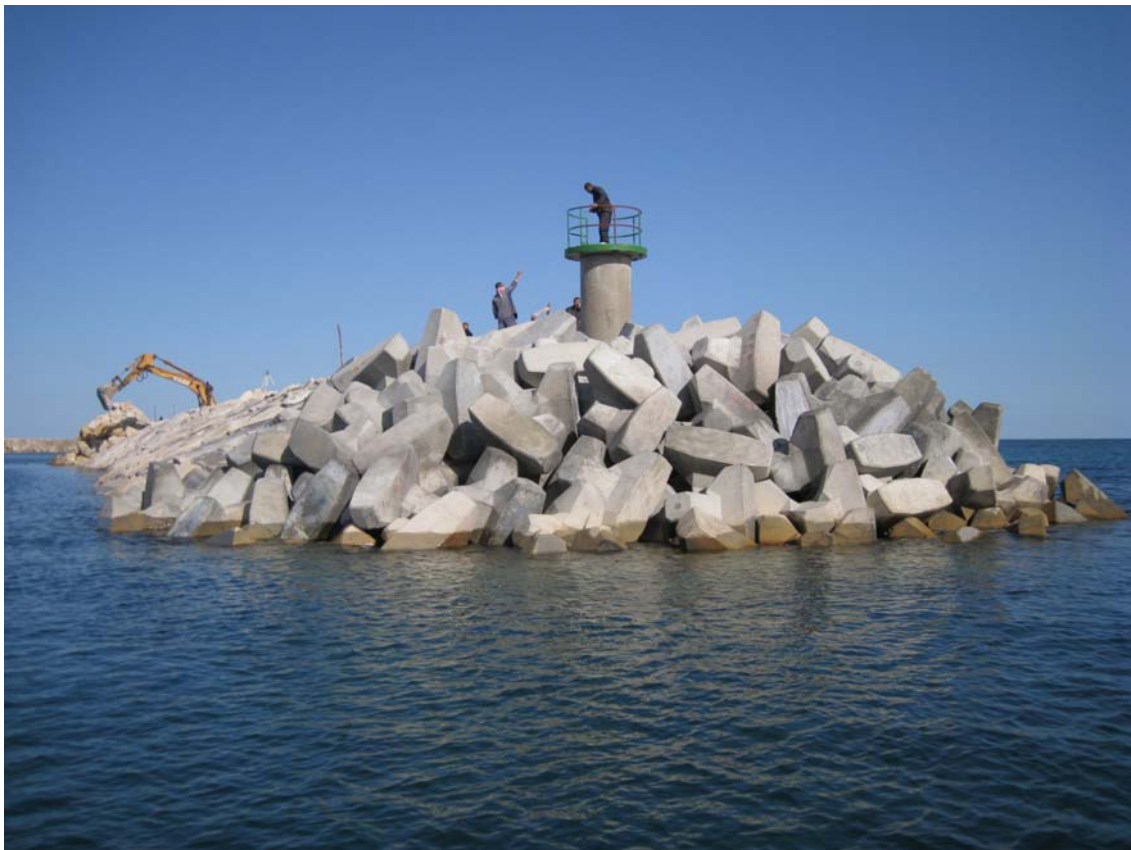
Photo no. 6 – Digue Nord – Musoir
