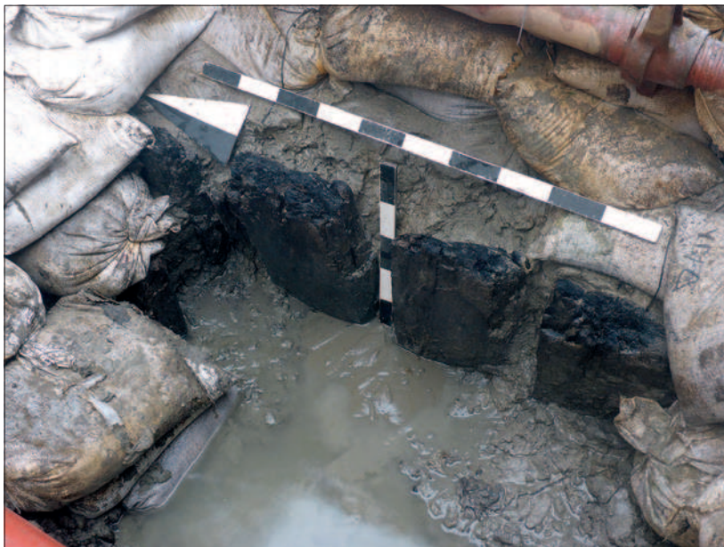
Fig. 12 Timbering of the canal fairway of the Fossa Carolina during the excavation 2013, dated to 793 AD. – (Photo L. Werther).
